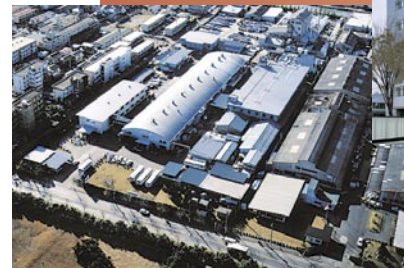
Soka Factory #1, New Building
